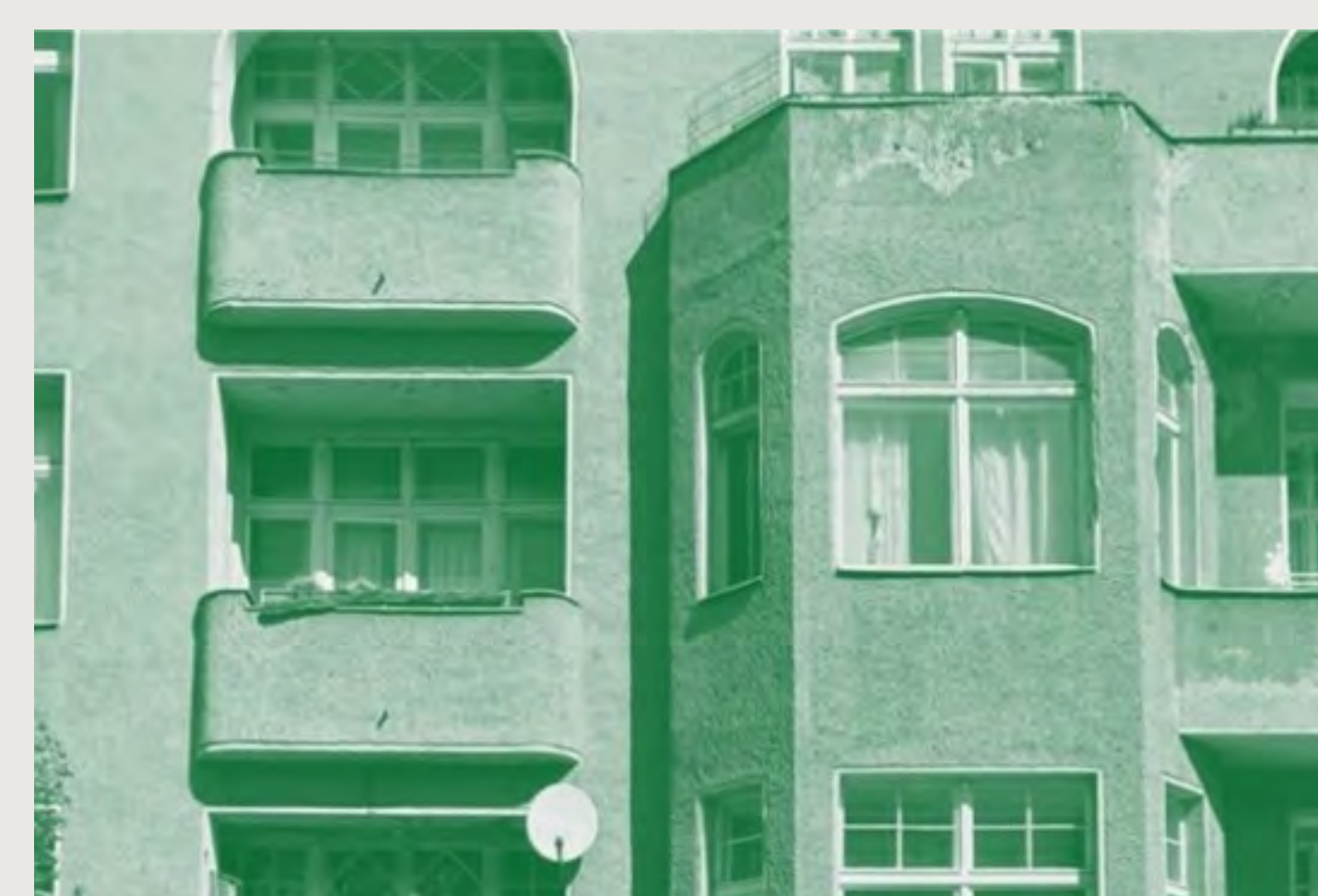
Typical Altbau urban Fabric and Construction. Image: Google Earth / Erhard
